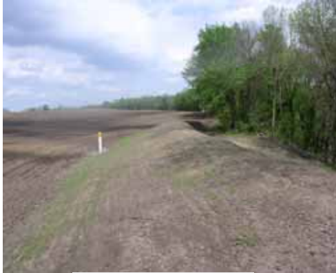
This is a completed Water & Sediment Control Basin project.
