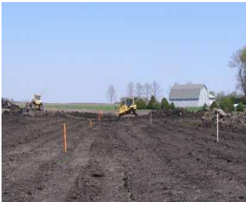
Waterway under construction
