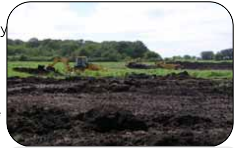
This drained wetland is being restored through a combination of tile breaks, sediment removal and earthen embankments.
