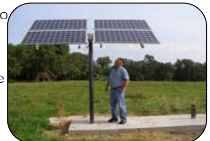
Paul - looking at the solar panel that produces power for his well pump.
