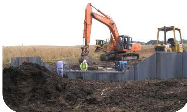
Cutting and shaping top for cap installation.
