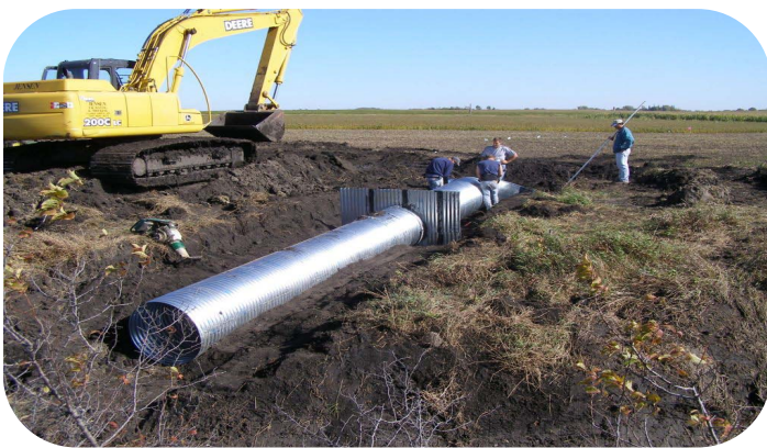
Pipe assembled and ready for backfilling.
