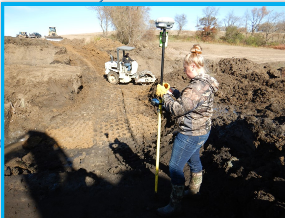
Resource Conservationist, Lindsey Zeitler surveying the core trench of the County Ditch 8 project.
