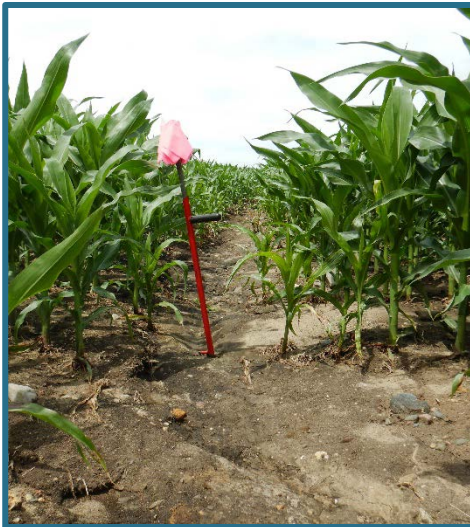
Flag holder showing the extent of the resource concern. A waterway will help reduce the erosion occurring at this site.
