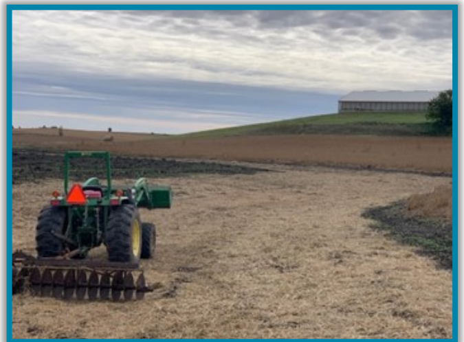
Preparing to crimp the mulch laid on a constructed Grassed Waterway to ensure establishment.
