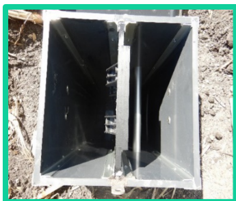
A controlled drainage system with all the boards
